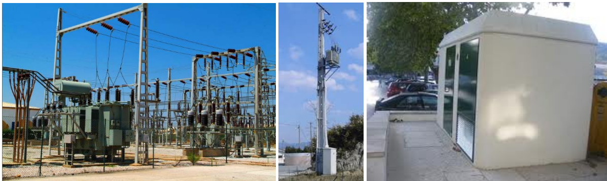
Figure 5 – Electrical substation (left) and distribution transformers (center and right)
