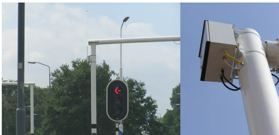
Figure 13: Example of a roadside unit at signalized intersection
