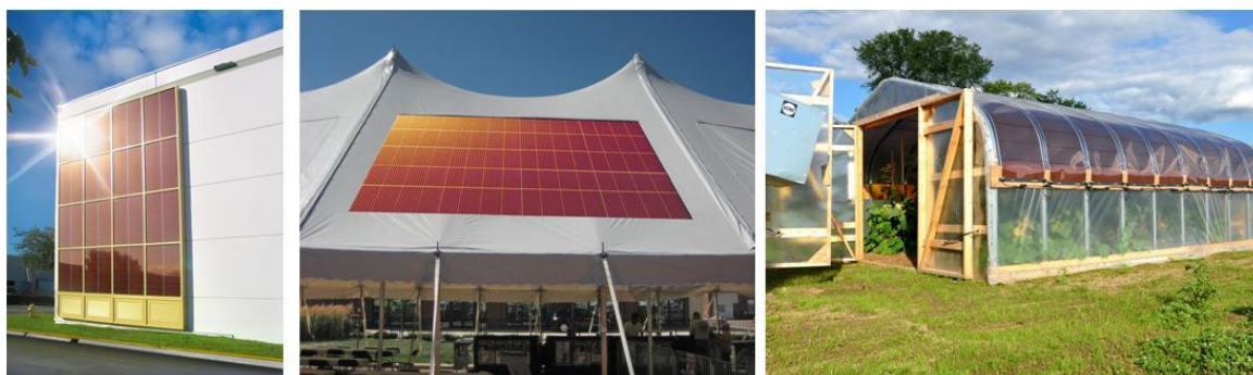
Figure 1. Examples of Large area demonstrations utilizing OPV panels. Left: curtain wall with OPV behind glass. Middle: OPV integrated in a shading structure providing both power and natural colling. Right: semitransparent OPV integrated in a greenhouse (Courtesy: Konarka),
