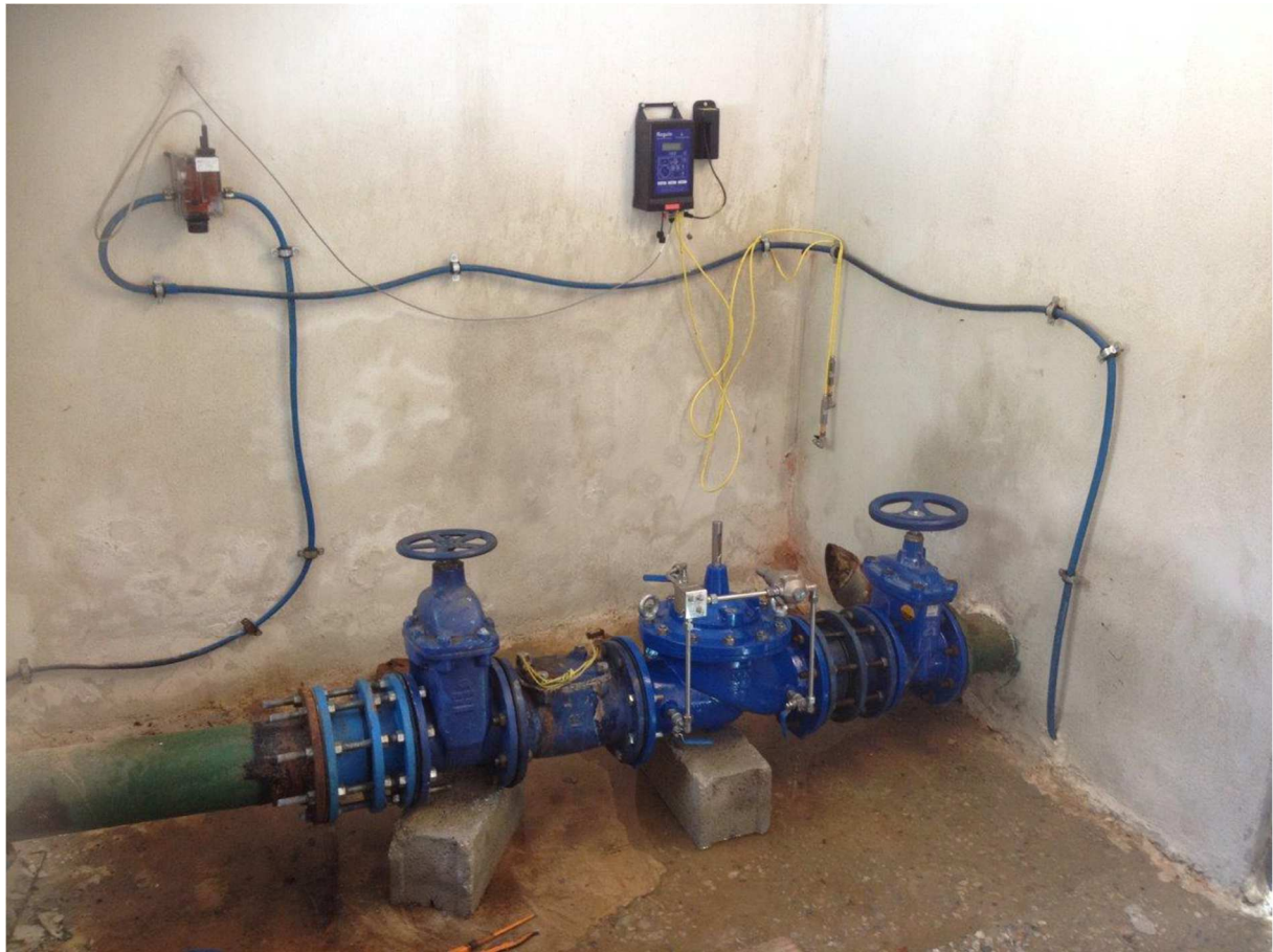
Figure 16. The PRV installed in Skiathos, completing the installation of urban-level equipment for both case studies.
