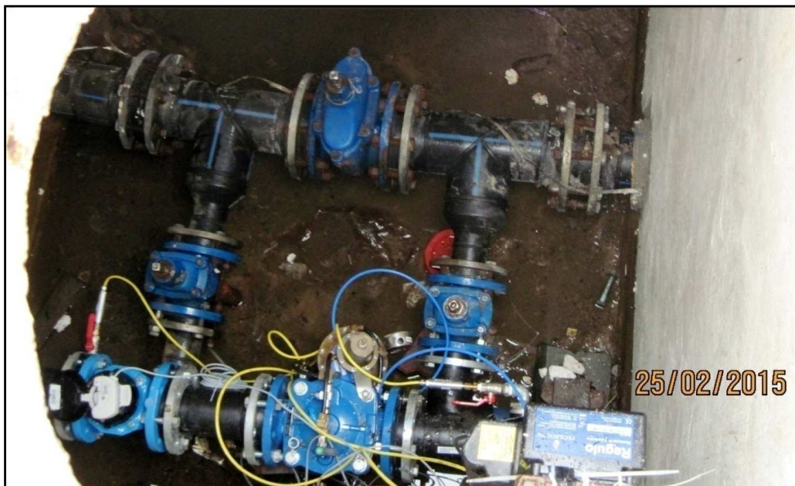
Figure 6. Equipment (water meter and PRV) installed in the 'Kolonia Cieśle' district
