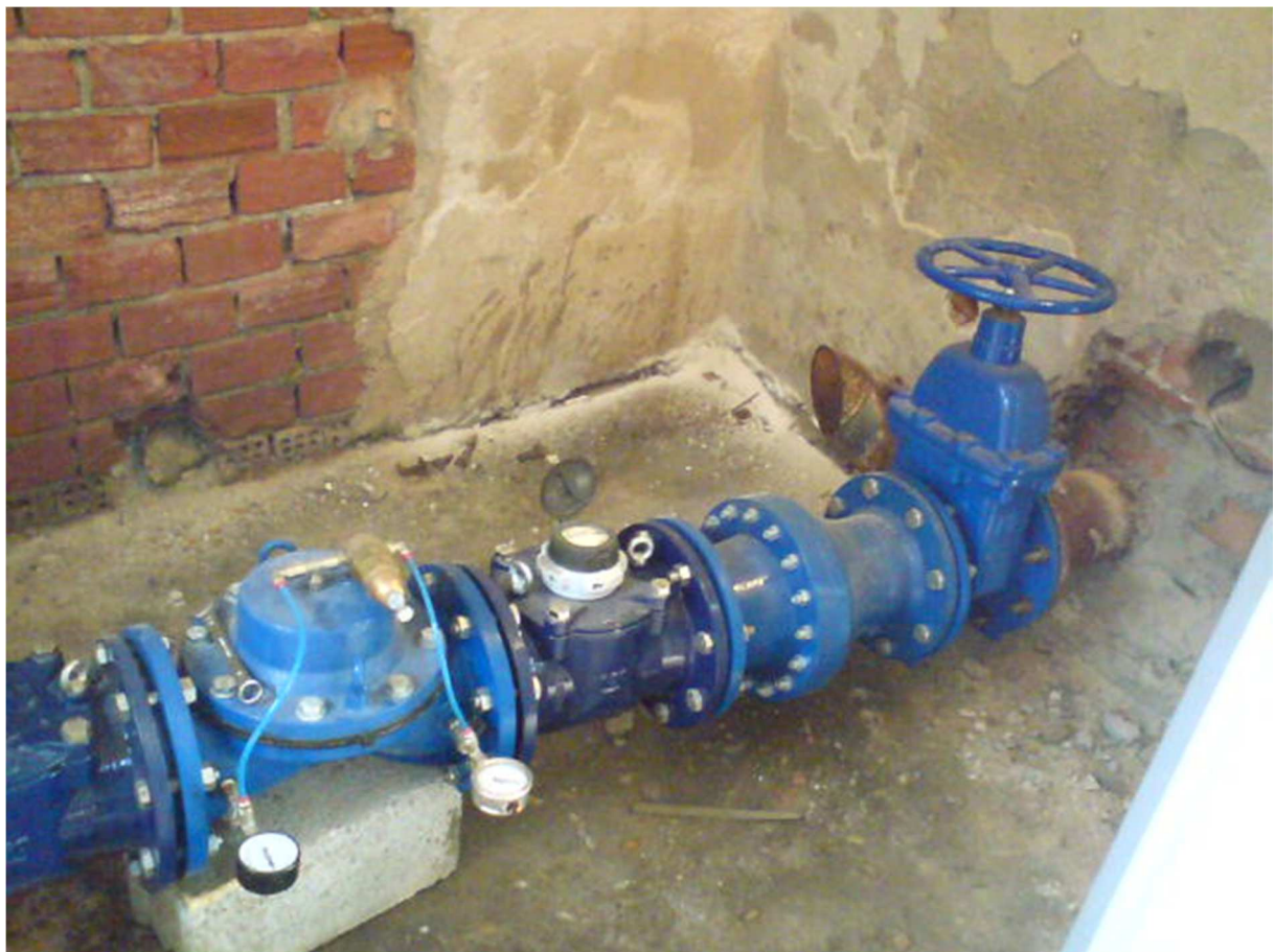
Figure 13. Example of the current setup of the pressure reduction in Skiathos
