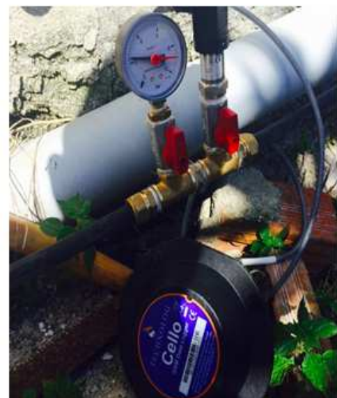
Figure 15. Installation of pressure control and pressure monitoring equipment in 3 critical points system at Skiathos Island.
