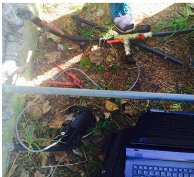
Figure 15. Installation of pressure control and pressure monitoring equipment in 3 critical points system at Skiathos Island.
