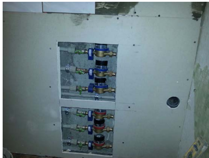
Figure 3: Apator monitoring system installed inside a wall
