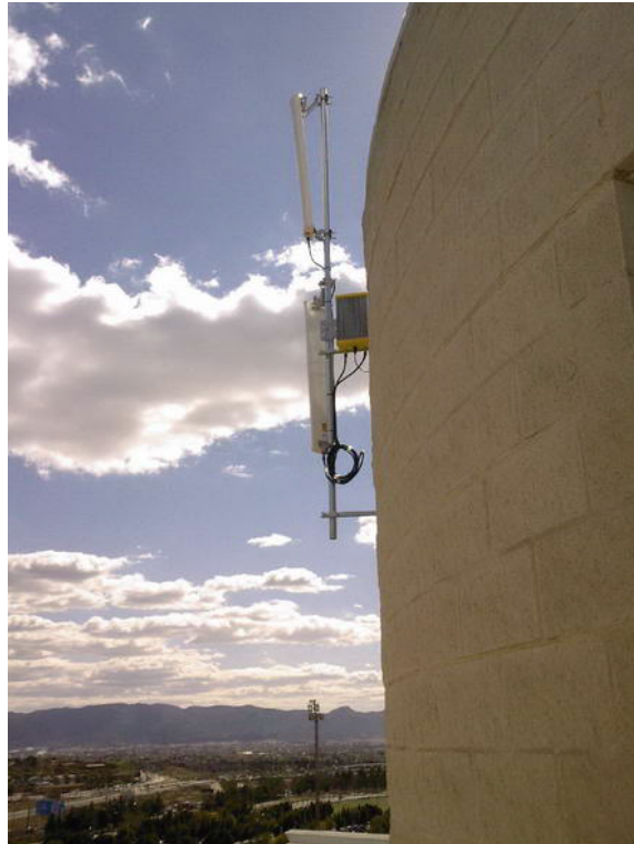
Figure 5.2: Access point used to provide 802.11b connectivity
