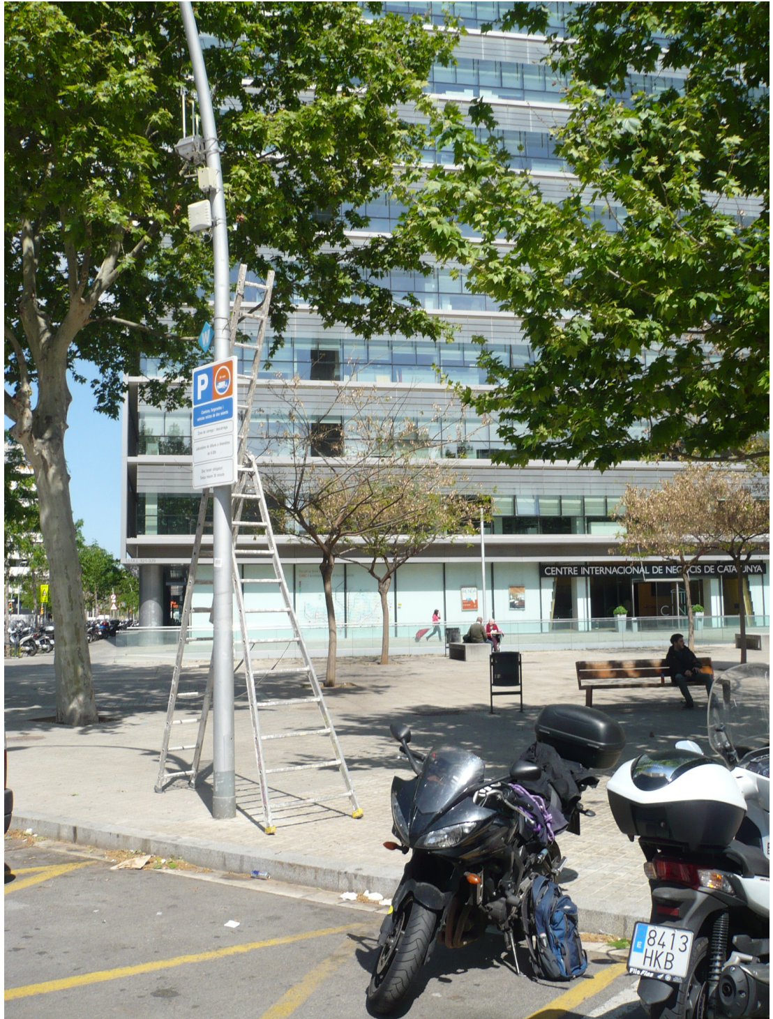
Figure 6: Picture of the base station with the border router (inside the white box) in the light pole.
