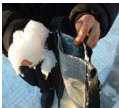
Fig. D36-17: Introduction of sorbents into the sockets
