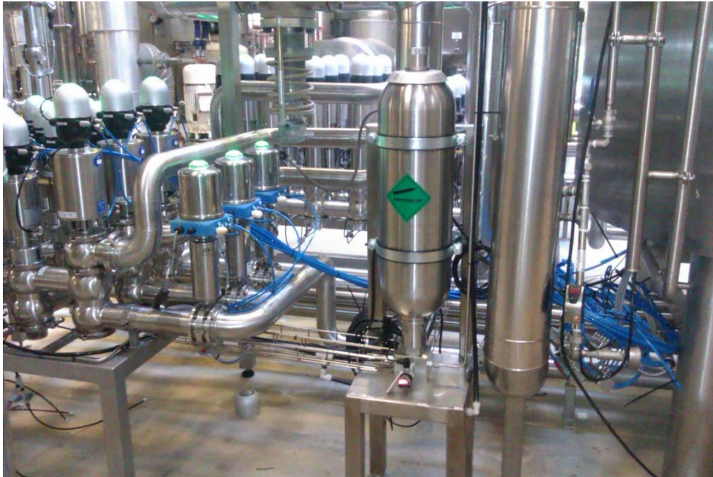
Figure 26. Hydraulic accumulator local to valve matrix
