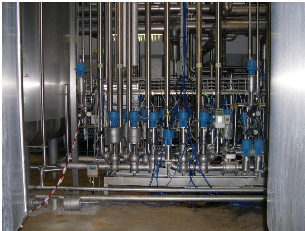
Figure 19. Pre-demonstration Hydract actuators fitted to GEA valves
