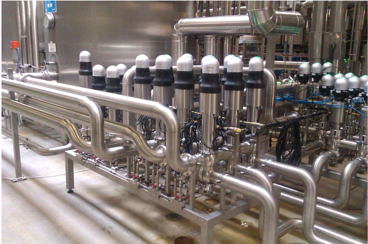
Figure 27. Matrix of 19 Hydractdem actuators in the forward valve matrix of CIP 2
