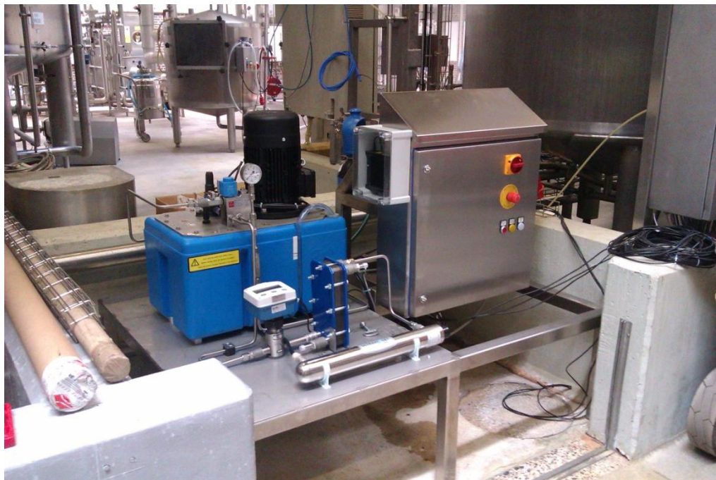
Figure 25. Hydraulic power unit for CIP 2 hydraulic valve actuators
