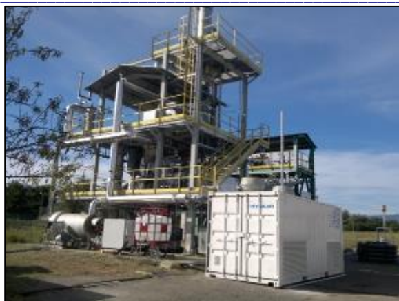
Figure_ 1 UNIfHY 1000 kWth gasifier with the PPS
