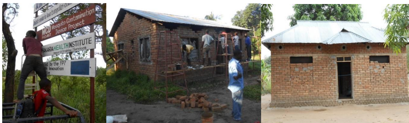
Fig. 11. Installation of eave tubes in local houses in Mngeta, Tanzania. A local team of constructors was trained to render houses mosquito-proof, which includes sealing openings (at wall/roof level) with bricks/cement, screening windows with untreated netting, and installing eave tubes.
