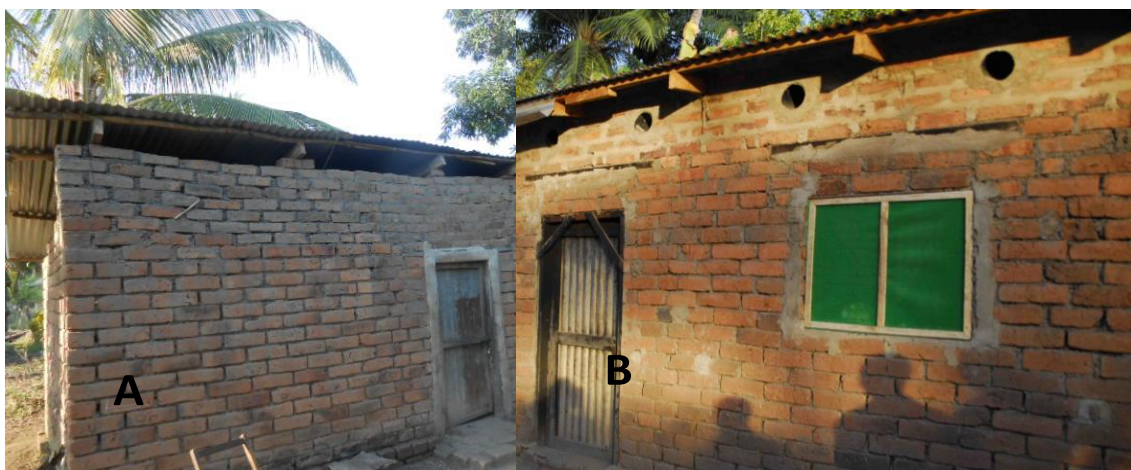
Fig. 14. Mosquito trapping studies were done in unmodified houses with open eaves (left) and houses in which eaves were sealed and eave tubes were installed with either untreated or insecticide-treated netting (right). Eave tube installations resulted in large reductions in indoor numbers of mosquitoes.
