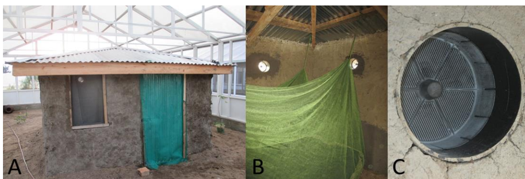
Fig. 8. Experimental house inside the Kenyan semi-field screenhouse (A), indoor view of eave tubes (B), and insecticide-treated eave tube, view from outside the house (C).
