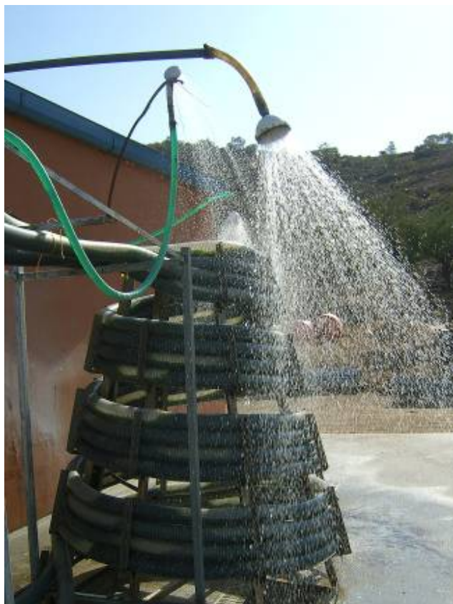
External shower cooling.
