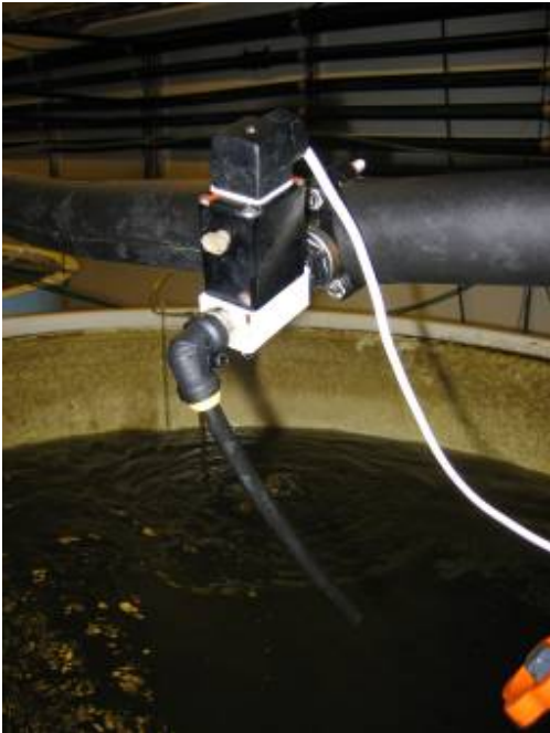
Example of an electronically controlled solenoid valve at SagFjord
