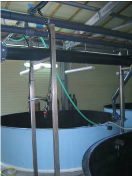
Larvae tanks with live algae distribution system.
