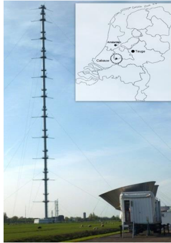
Figure 4: Picture of the 213 metre high mast in Cabauw, hosting different meteorological remote sensing instruments, including IDRA, a, X band polarimetric radar. On the internal square, displacement of Teuge and of Cabauw site.
