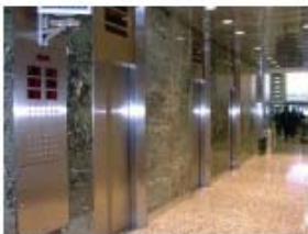
Turn off 1 of 4 elevators
