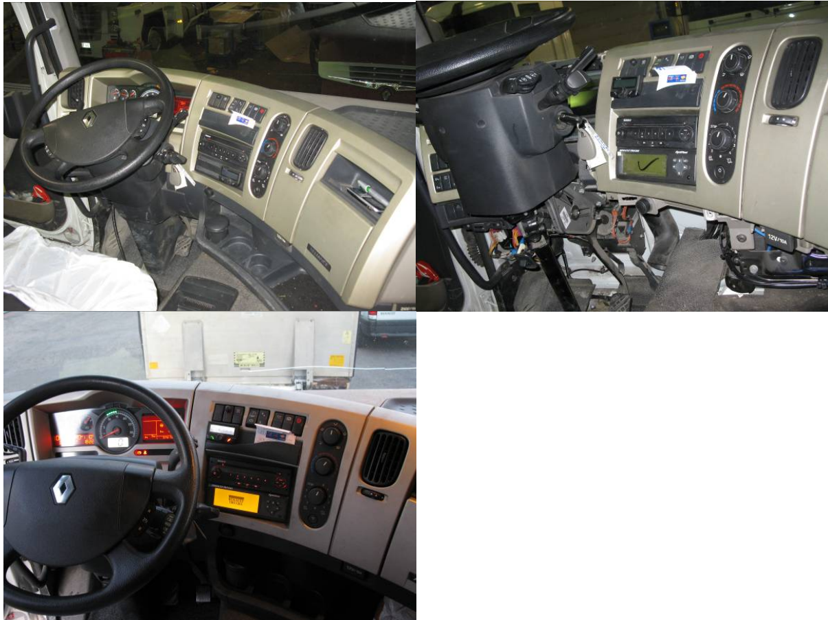
Figure 32: Driver cabin from before (top left), during (top right) and after (bottom left) installations
