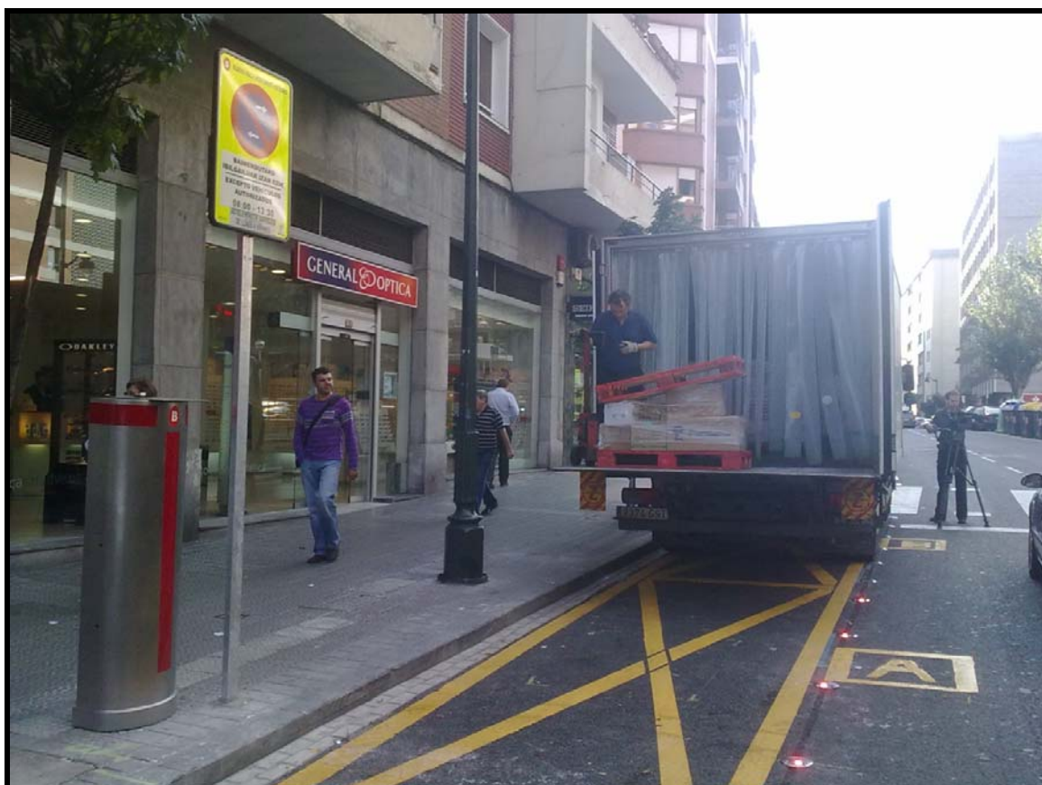
Figure 26: Trucks proceeding with the download operation
