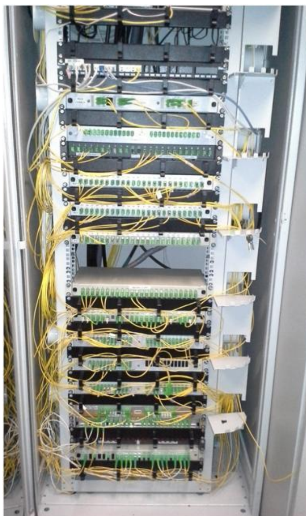
Figure 9: Main building ODF
