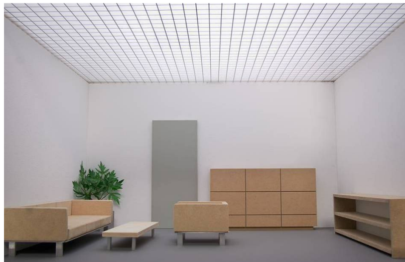
Fig. 3.24: Living room model with an OLED ceiling luminance of 300 cd/m 2 , OLED tile size is 15 x 15 cm 2
