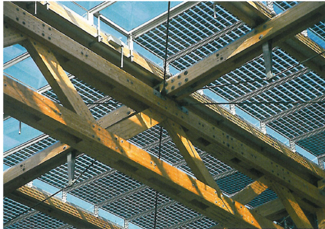
Fig. 3.6: Integrated solar module on the glass shell construction of the Academy for Further Education, Herne, 1998, Arch.: Jourda & Perraudin Architects with HHS Planer
