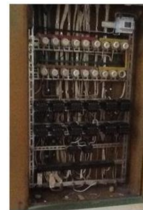
Figure 2-31: Installed smart electricity meter in Floor sub-distribution board 2
