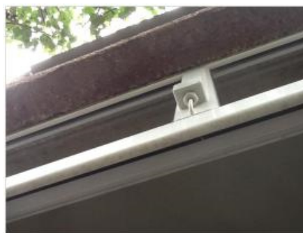
Figure 2-28: External temperature sensor installed on the exterior window of the Corridor 1
