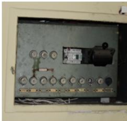
Figure 2-30: Installed smart electricity meter in Floor sub-distribution board 1
