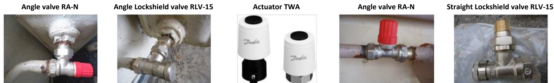
Figure 2-26: Pictures of installed valves in Plovdiv
