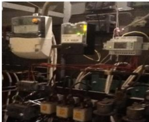
Figure 2-29: Installed smart electricity meter in Main distribution board 1
