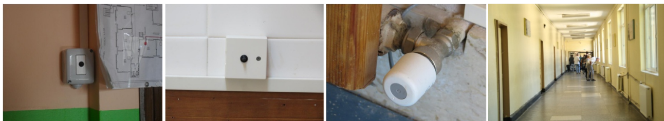
Figure 3-9: Temperature sensors and ON/OFF valve on radiators.
