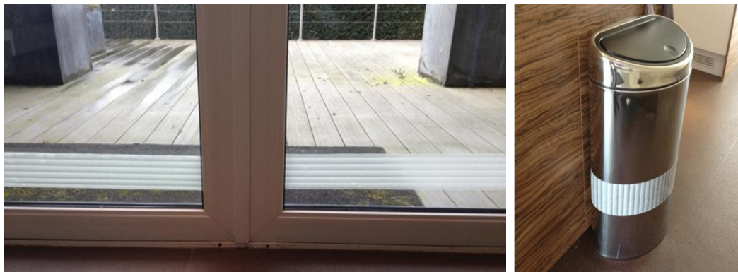
Figure 44 a temporary solution to low windows and reflections: white tape
