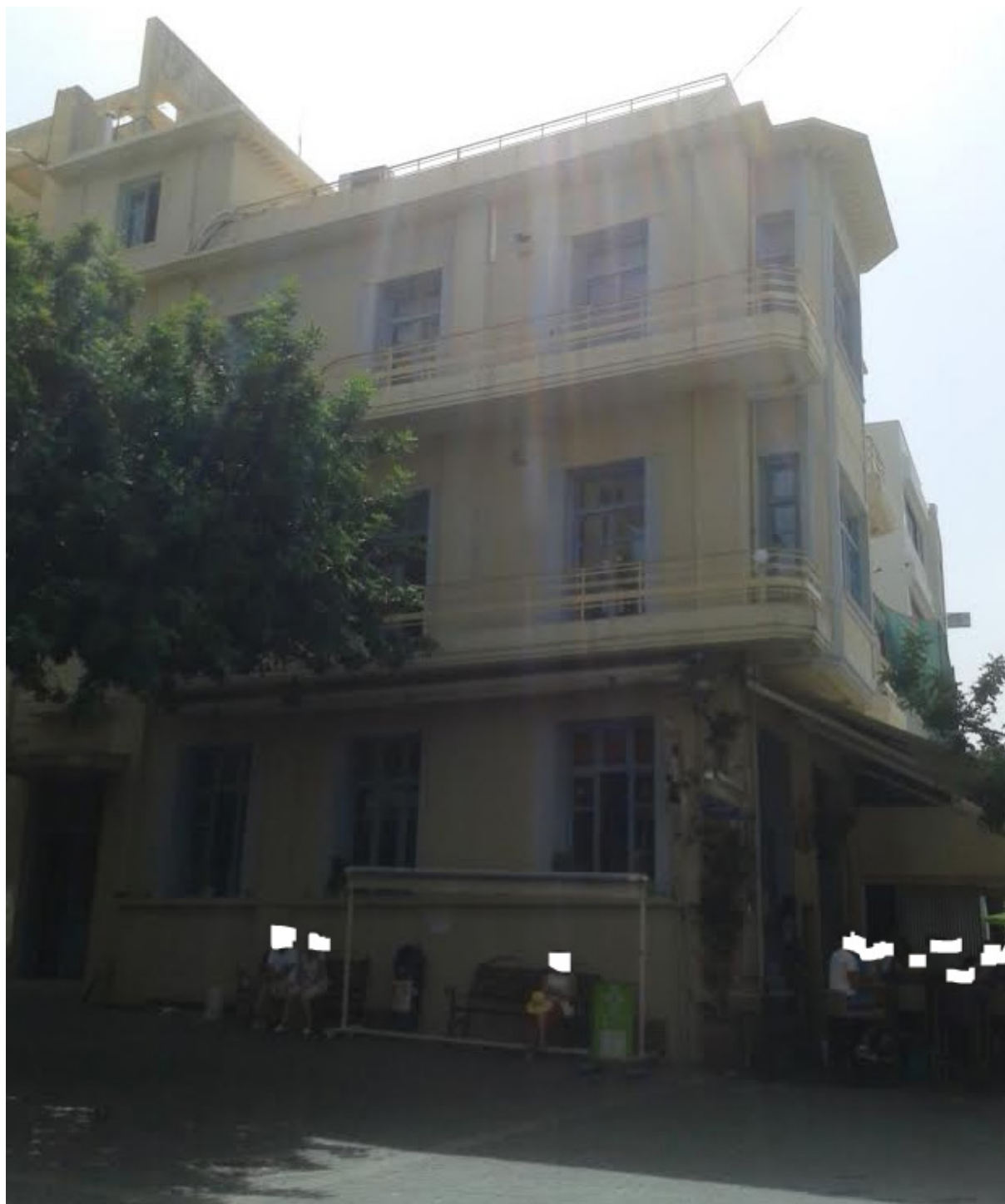
Figure 22 The building at Androgeo
