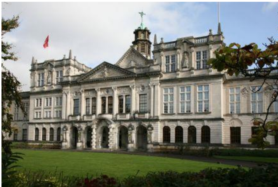
Figure 1 - Cardiff University Main Building
