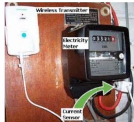
Picture 19: Meter installation for Smart metering project
