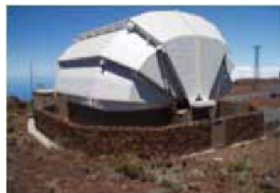
Figure 3. The enclosure for Faulkes Telescope North
