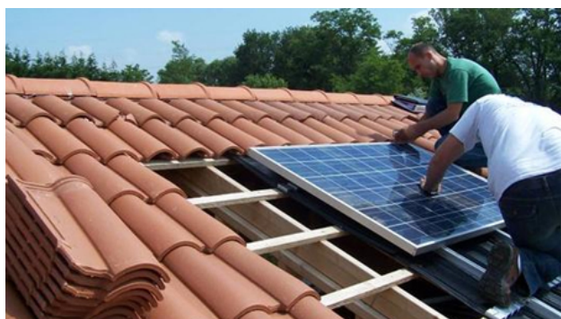
Figure 13 - PV Full-building integration
