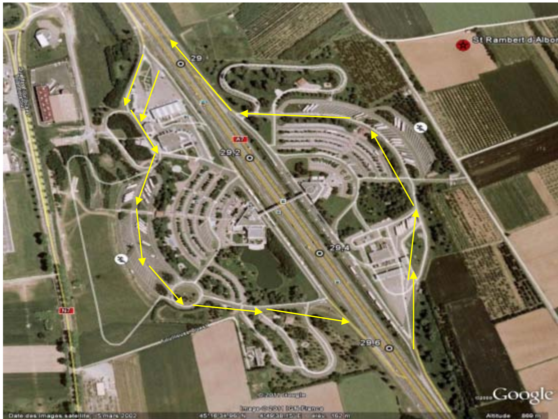
Figure 32 - Saint Rambert d'Albon east and west (A7 motorway)
