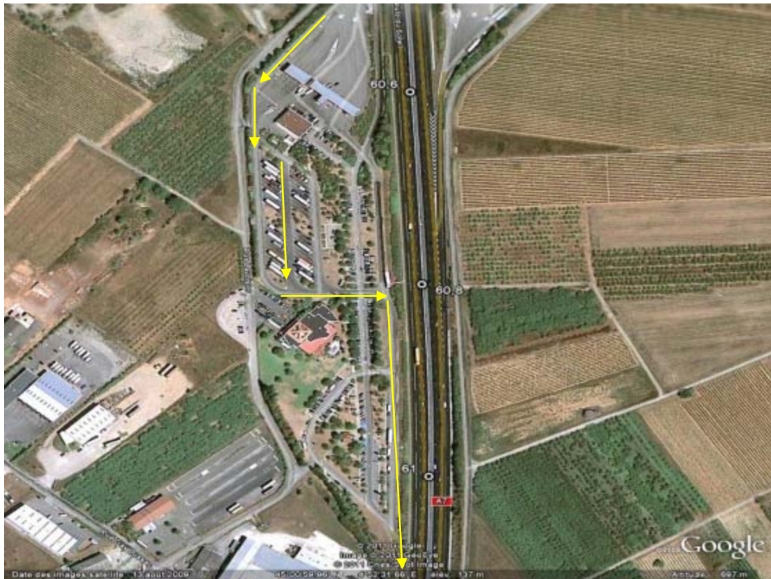
Figure 34 - Pond d'Isère, (A7 Motorway)
