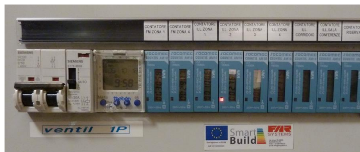
Figure 6. All pilot buildings were comprised with numerous sensors to measure energy streams and comfort parameters within the building. This picture shows electricity meters installed to monitor electricity flows on branch level.
