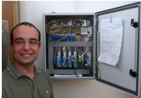
Figure 7. ICT data are collected in central electric cabinets on room, zone and/or floor level. The web based “FAREcho energy portal” connects to the central electric cabinet of any building.
