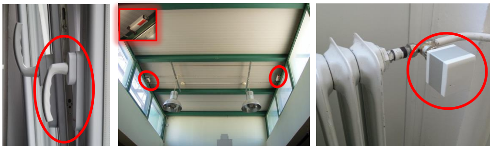
Figure 8. Selection of ICT technologies implemented, including for cutting edge wireless electronic thermostatic radiator valves, eTRVs, using energy harvesting technology (picture to the right).
