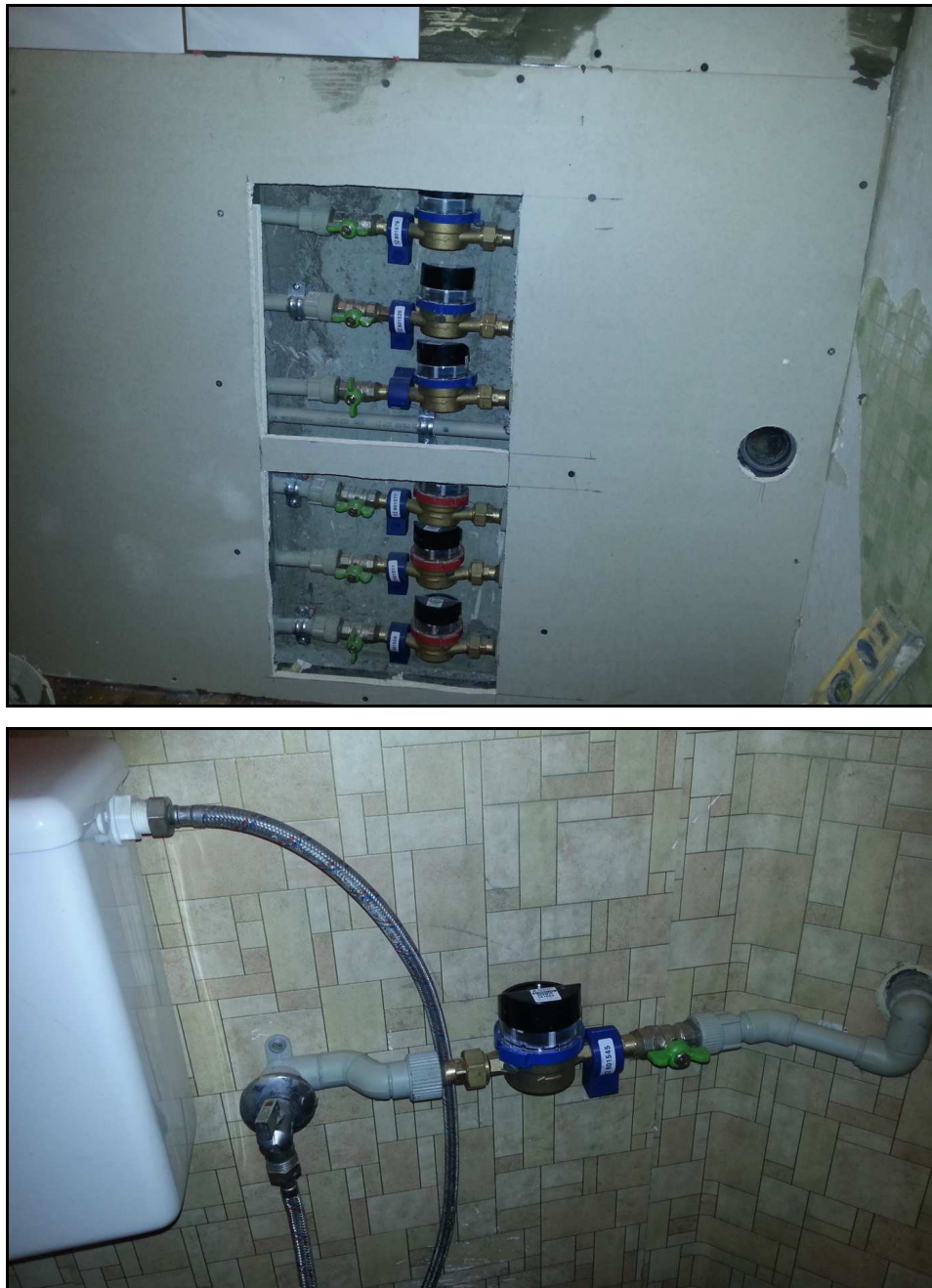
Figure 17. Top: Six water meters monitoring hot and cold water (kitchen tap, bathtub tap and bathroom tap); bottom: Water meter mounted on the toilet flush
