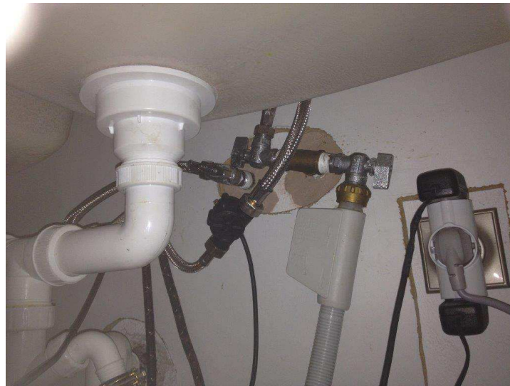
Figure 19. One flow/temperature sensor is installed with the water supply pipes
