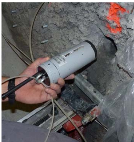
Figure 8: Detail of node installation.
