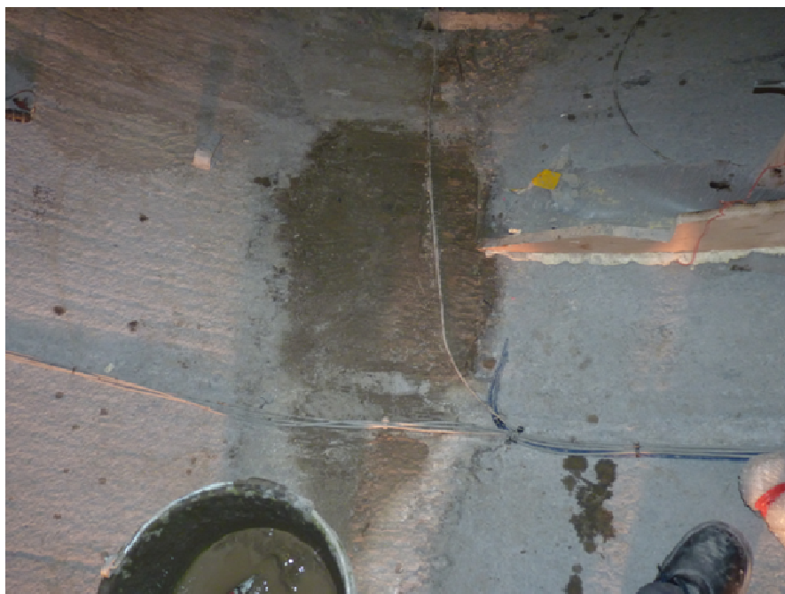
Figure 9: Detail of node installation.
