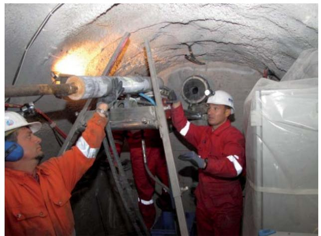
Figure 5. Drilling through the 2.2 m thick concrete plug into the bentonite for core sample extraction.
