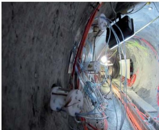
Figure 1. Three piezoelectric transducers just after installation close to the tunnel wall. These were covered later by the sand-bentonite mixture.
