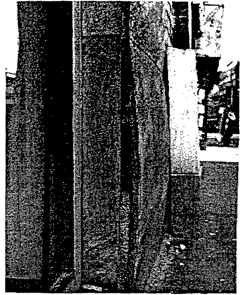
Fig.2. Bowed panels of fine grained marble in Vienna
