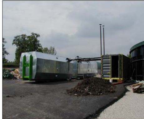
Figure 3: View on the 3A-biogas testing plant
