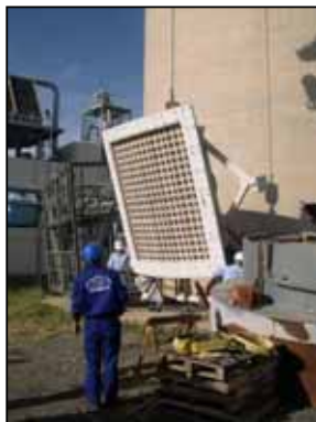
Figure 1.2-13: Lifting of SOLAIR receiver steel structure on tower
