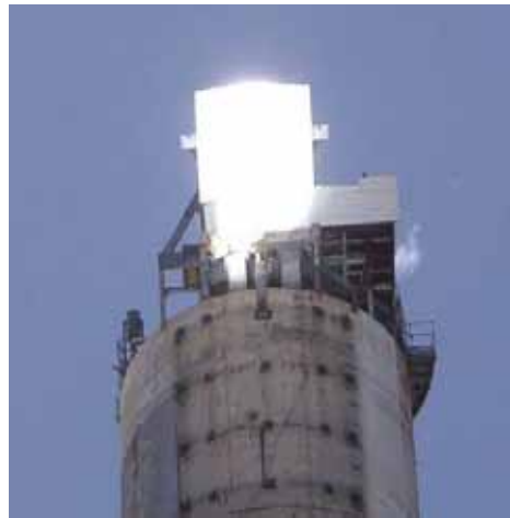
Figure 1.2-17: 3 MW receiver in operation
