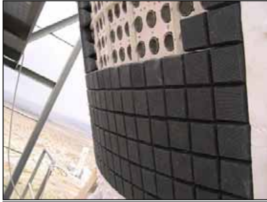
Figure 1.2-14: Mounting ceramic absorber modules
