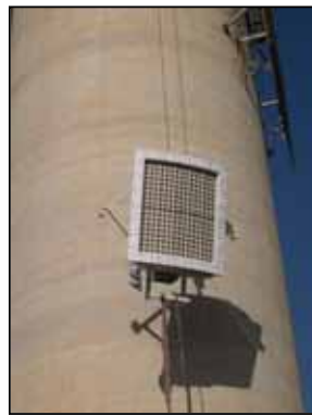
Figure 1.2-13: Lifting of SOLAIR receiver steel structure on tower
