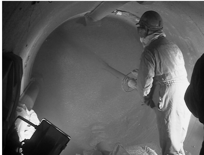
Figure 5: Construction of second section of the plug
