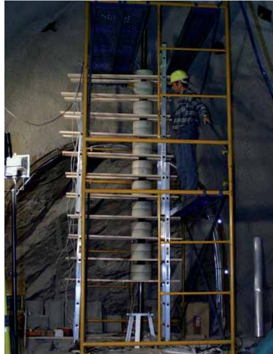
Figure 2.4: Detail of the heater/buffer assembly installation.
