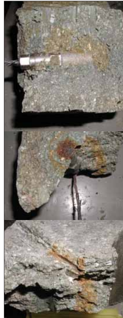
Figure 4.3: Details of corrosion of sensors in a bentonite block.
