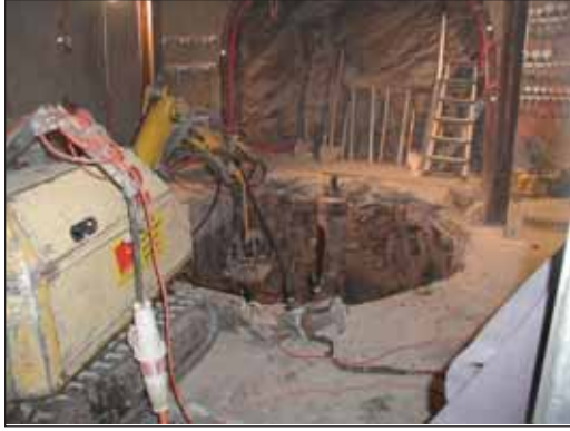
Figure 4.2: General view of the excavation work (phase 1).
