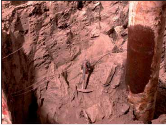
Figure 4.7: View towards the thrust zone between 0 and 2.5 m depth (view towards the rear end of the HE niche). A grid was installed for precise mapping. Right: the central heater borehole containing the heater casing.
