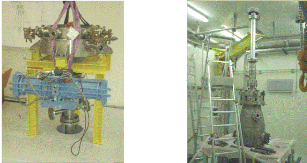
Fig. 32: KROTOS installation in the PLINIUS building extension
