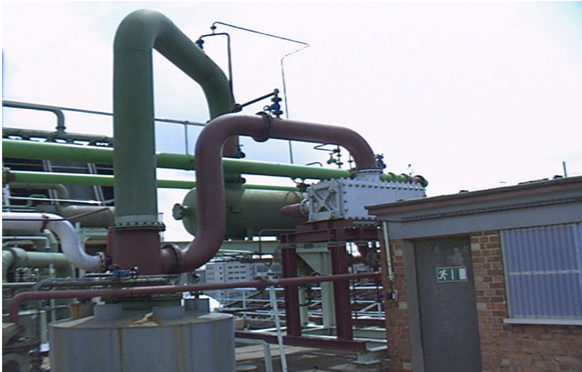
Figure 10: Integration of the downward condenser
