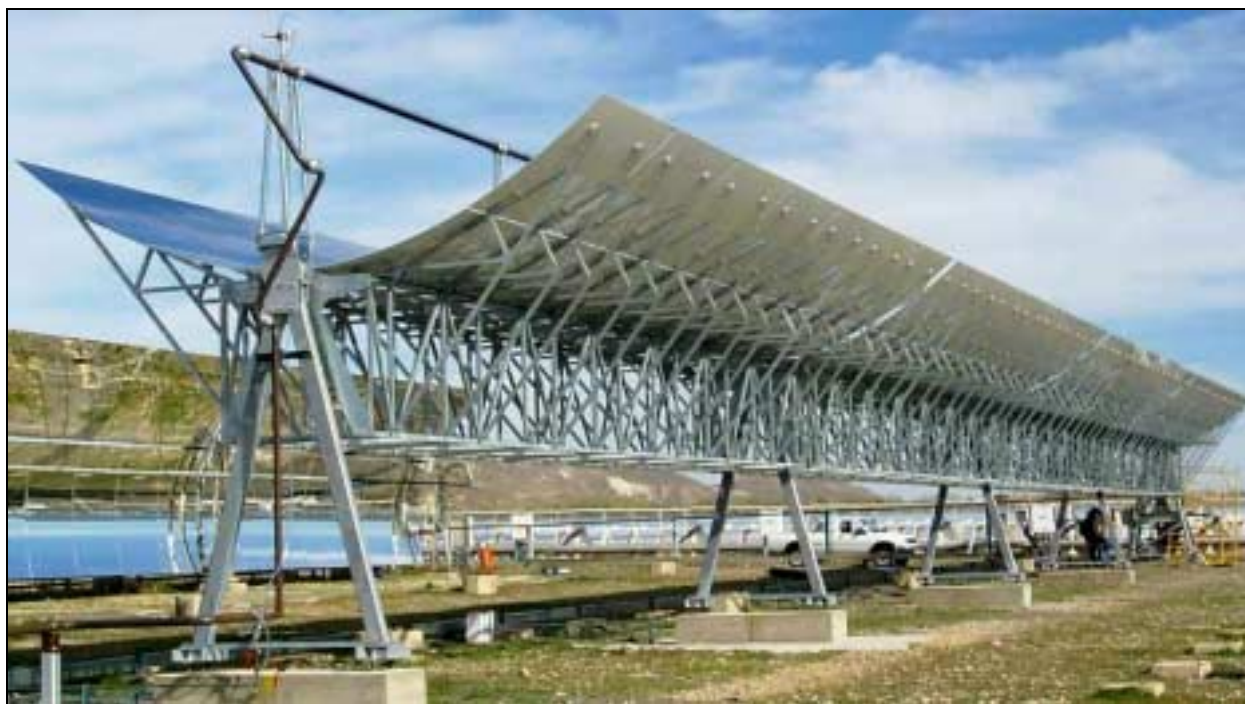
Figure 5 EUROTrough Prototype at the Plataforma Solar de Almería
