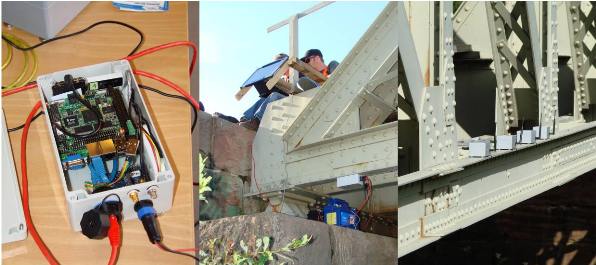
Figure 4. Wireless strain sensors used at the Keräsjokk Bridge close to the border between Sweden and Finland.
