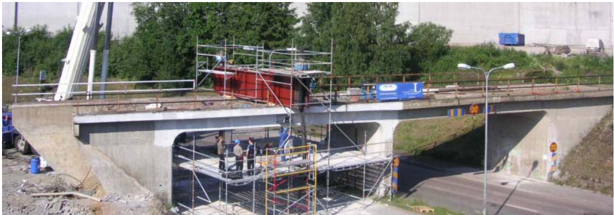
Figure 2: Automatic non-destructive testing (NDT) with radar and ultrasonic echo was used to check the concrete and reinforcement conditions in a redundant reinforced concrete bridge in Örnköldsvik, Sweden. The bridge was then tested to failure to compare assessment predictions with the real ultimate load-carrying capacity.
