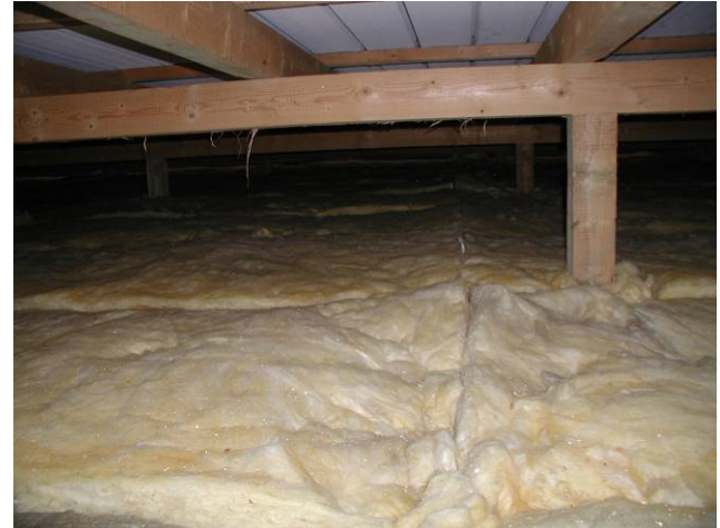
Figure 7.5: Although the construction is not well designed, because of ice and snow-free areas, there is no condensation inside because of the ventilation space of larger than 1 m. And such a wide space also could be found at other (renewed) roof constructions. This resulted in a recommendation for roofers to provide enough space for the ventilation and use roof area for solar elements. For the design the client has to have physical consultancy and suitable indoor ventilation.
