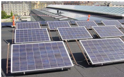
Figure 4.14: PVT panels where heat is fed to a heat pump in this way cooling the PV modules
