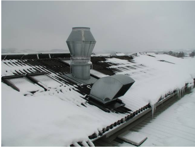
Figure 7.5: Although the construction is not well designed, because of ice and snow-free areas, there is no condensation inside because of the ventilation space of larger than 1 m. And such a wide space also could be found at other (renewed) roof constructions. This resulted in a recommendation for roofers to provide enough space for the ventilation and use roof area for solar elements. For the design the client has to have physical consultancy and suitable indoor ventilation.
