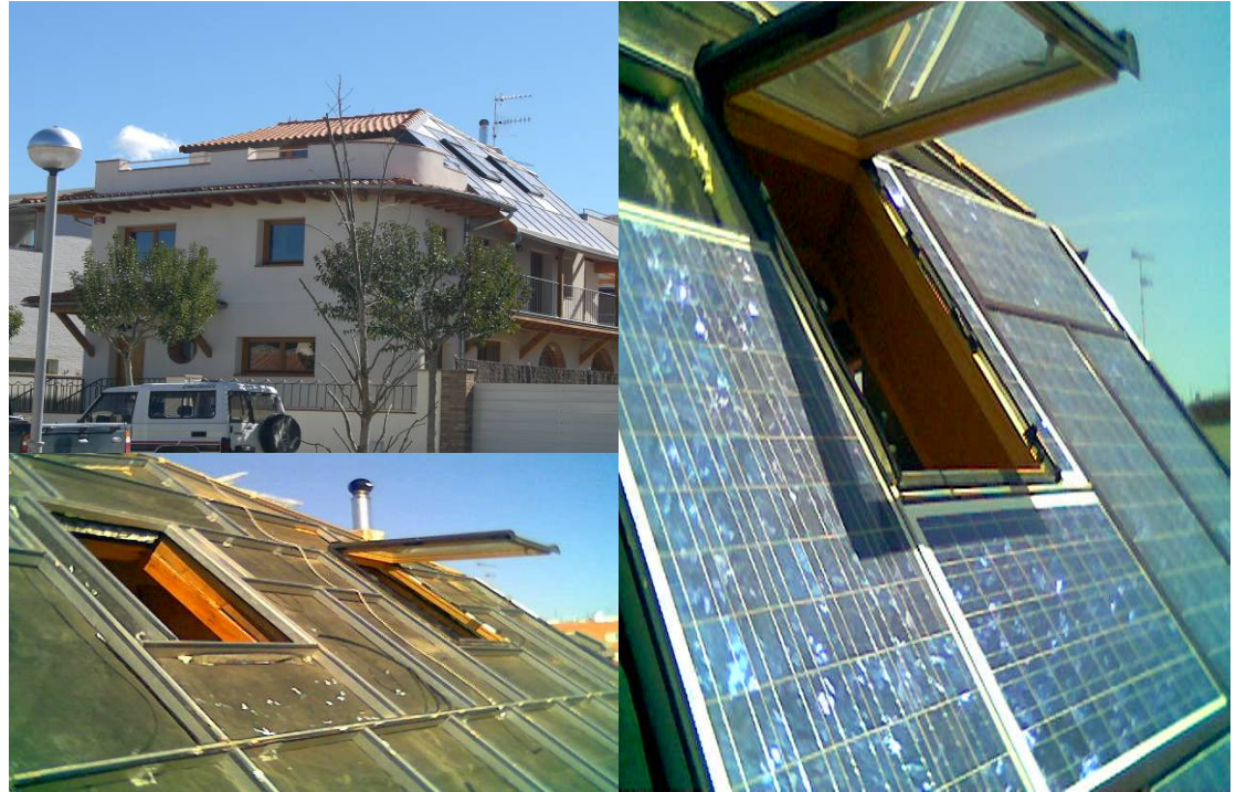
Figure 4.12: Illustration from full scale test in Spain with new type of roof integrated PV solution as substitution of old PV-installation of poor quality
