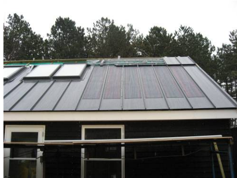
Figure 4.17: SOLTAG 2. Solution with innovative diffuse open Master Roof False roof solution with paper granulates insulation and a PVT solution in the roof which works in combination with a heat pump.
