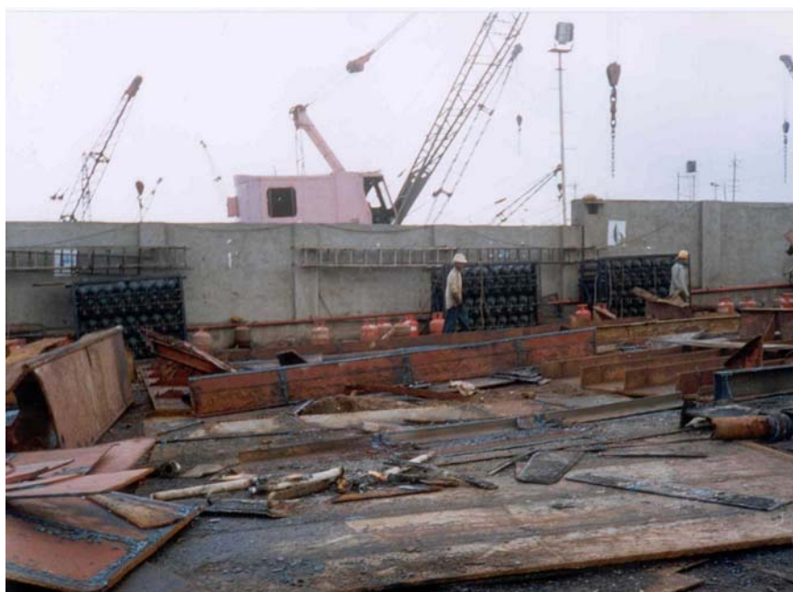
Figure 2.1: Steel plates recovered after dismantling of ship
