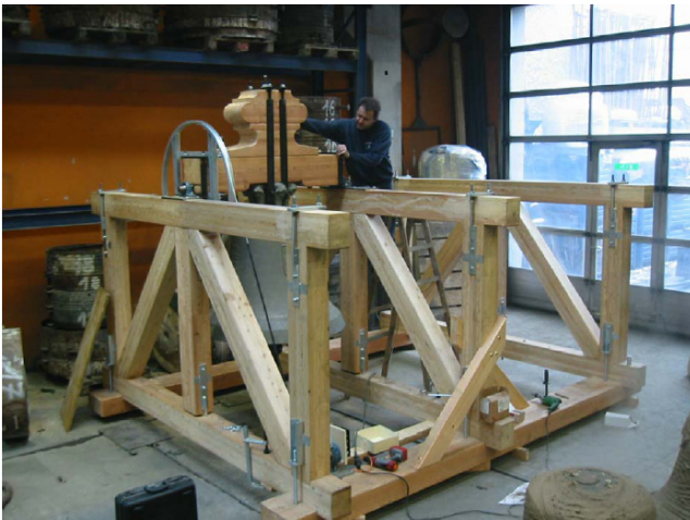
Fig. 8: Construction of PROBELL belfry for bells with 1to and 2,5to weight at Grassmayr
