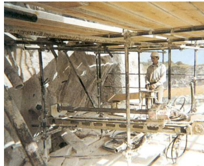
b) Drilling process on scaffolds
