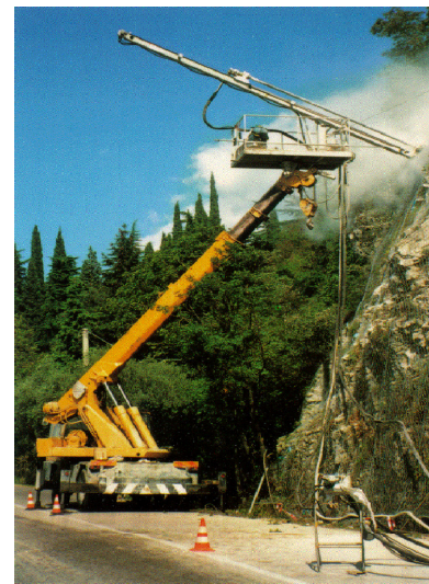
c) Drilling unit on board a crane
