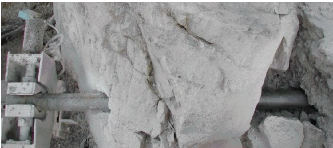
Figure 41: Void situation artificially generated during a test
