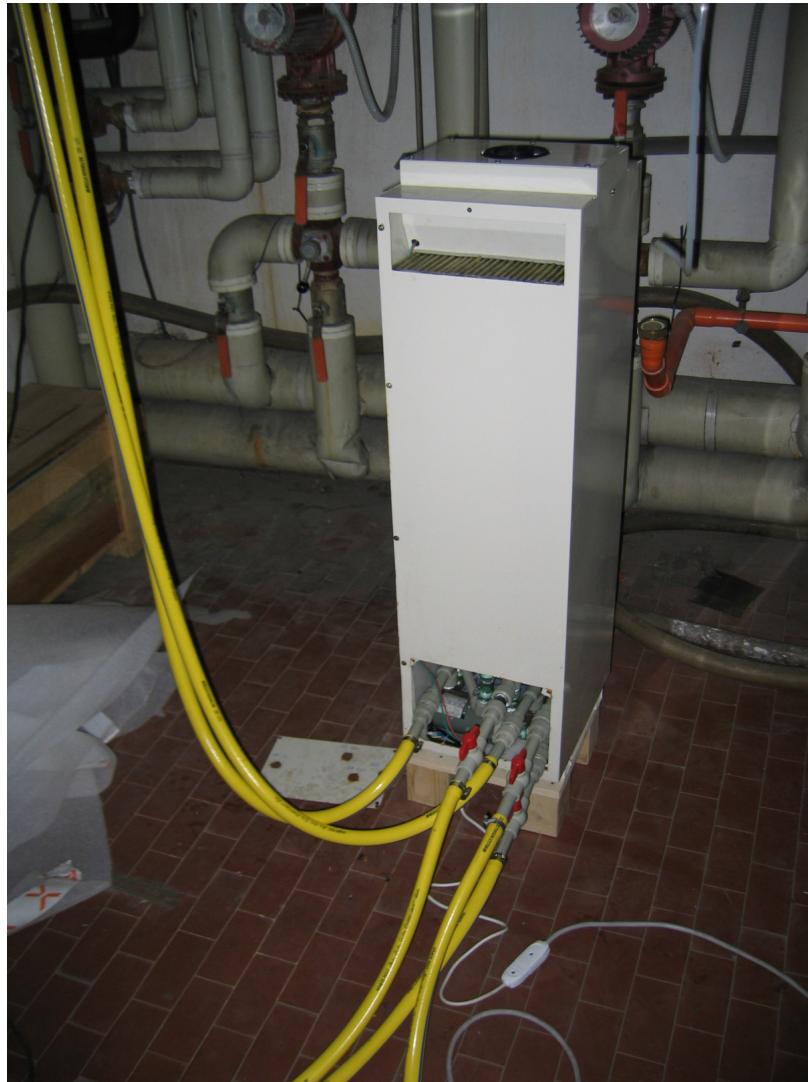
Figure 58: regenerator connected to hot water and central unit.
