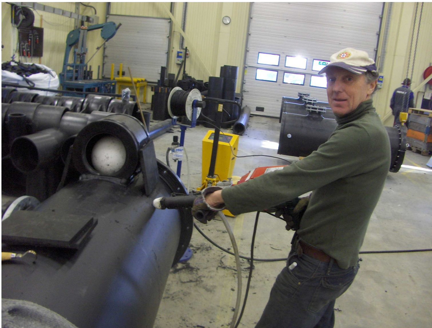
Figure 13 – Torger Tveter (IDEUTVIKLING) working on a pump
