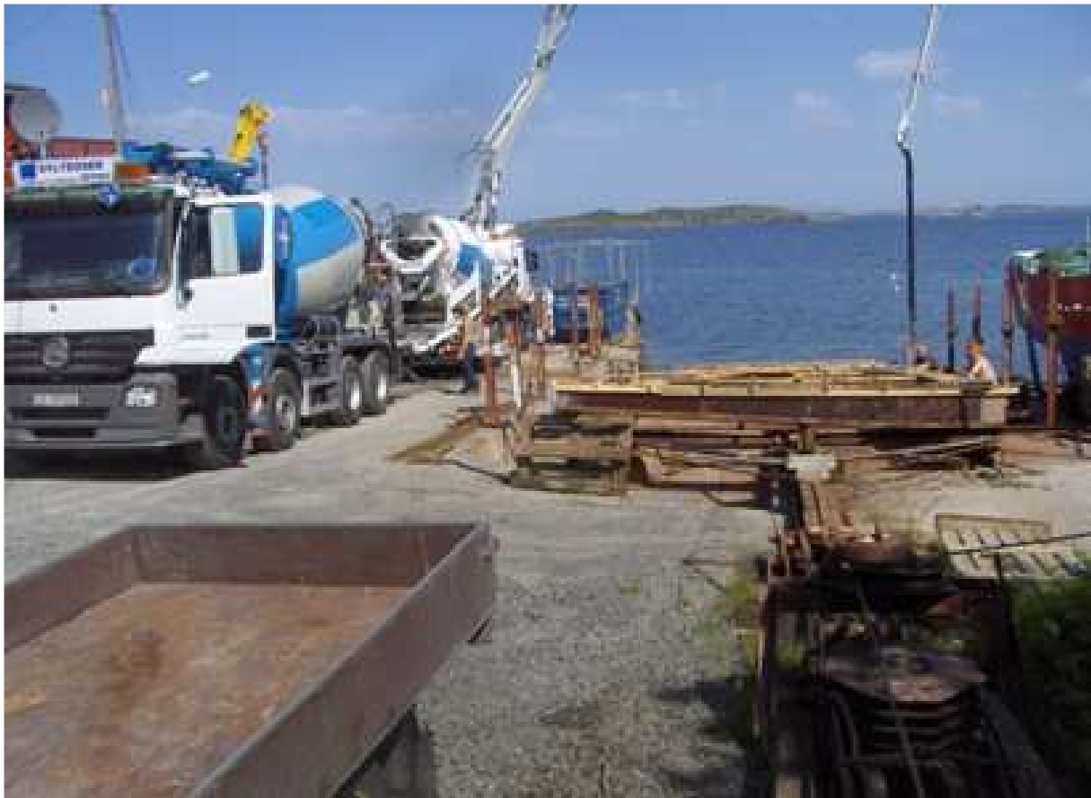
Figure 18 – The anchoring platform
