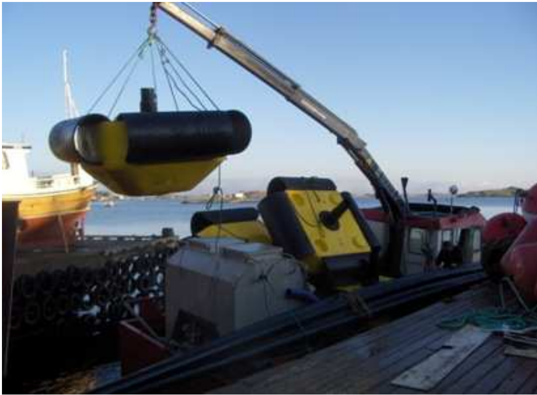
Figure 19 – Installation of the buoys
