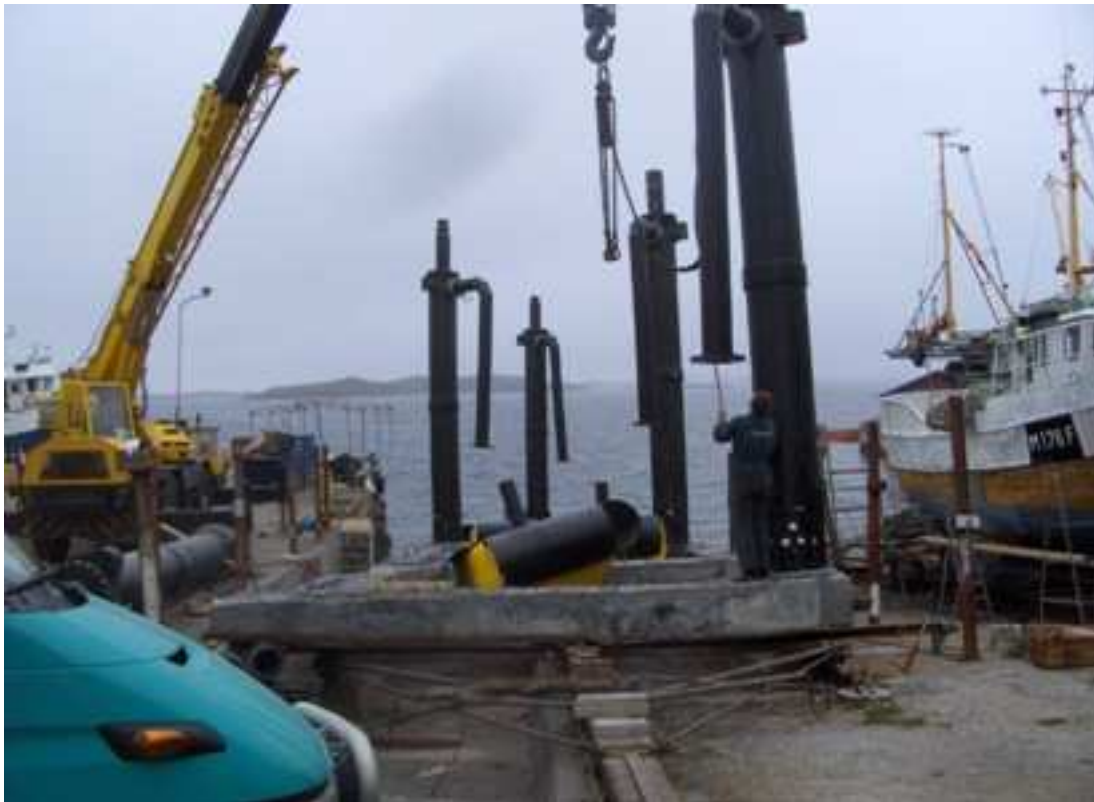
Figure 21 – Construction of the prototype
