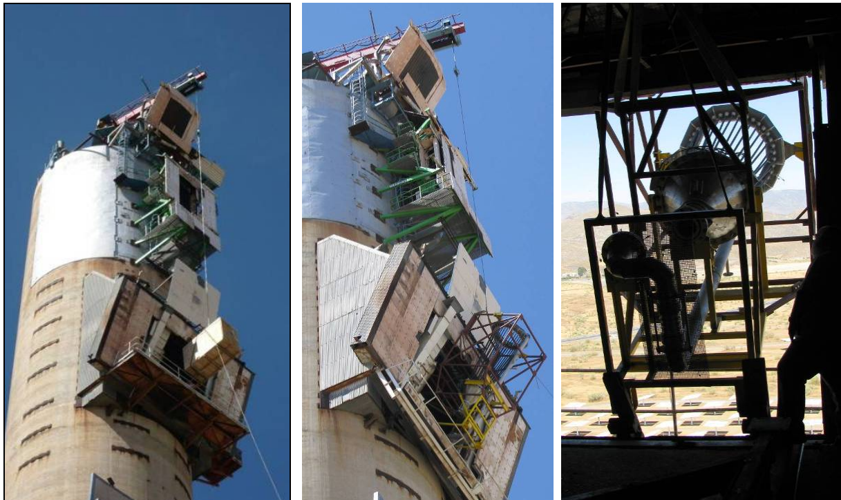
Figure 47 Lifting and installation of turbine and receiver
