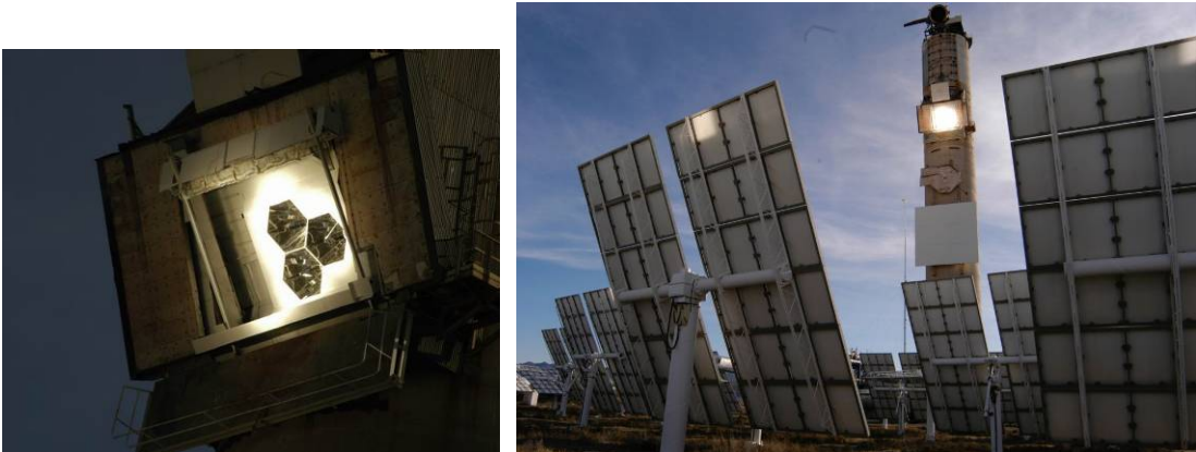
Figure 26 CESA-1 tower (r.) and detailed view on receivers (l.)
