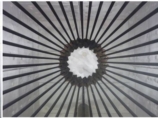
Figure 65 All sheets installed
