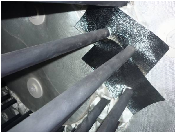
Figure 64 First Inconel sheets on back side of cavity installed
