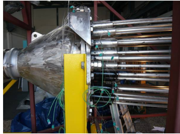
Figure 41 Installation of thermocouples
