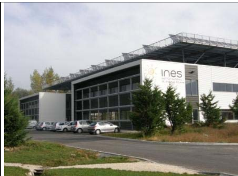
Figure 7 – PV array of Ines facility
