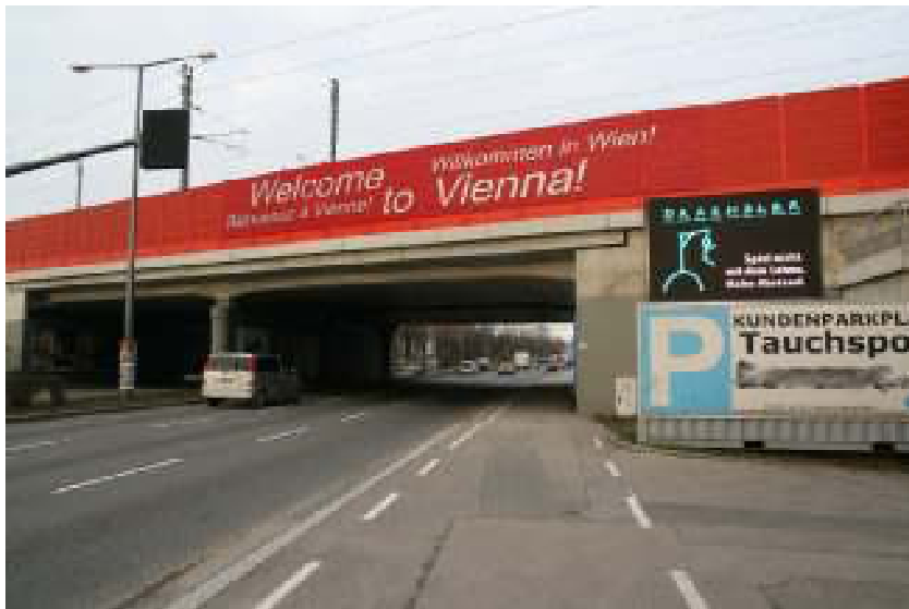
Videowall sign installed on one of the main entrances to Vienna
