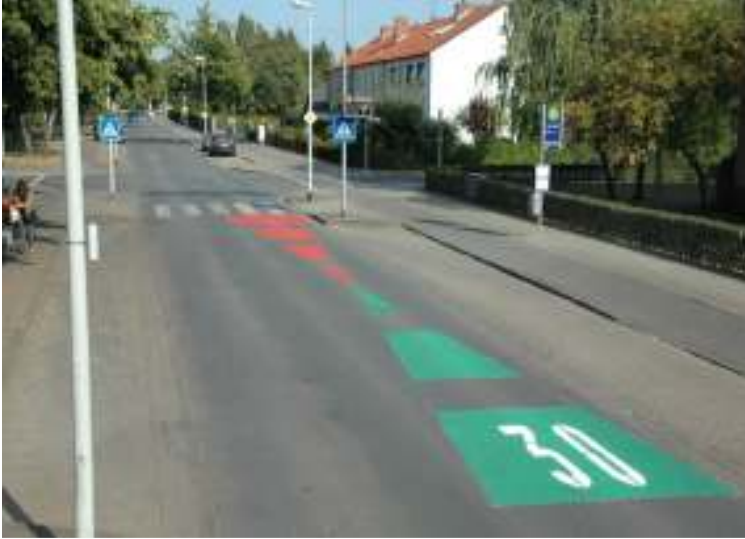
Implementation of special road painting in Hannover in a 30 km/h speed limit road
