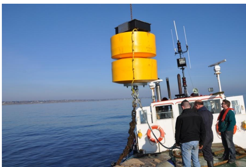
Figure 3.23: Mooring Buoy being deployed at Galway Bay Test Site
