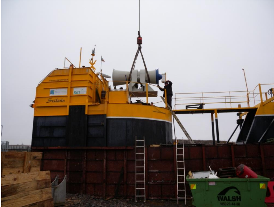
Figure 3.2: Installation of CORES Air Turbine onboard OE Buoy
