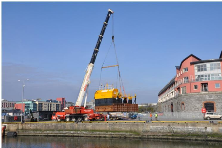
Figure 3.6: 100T crane lifting OE Buoy into the water in Galway Harbour
