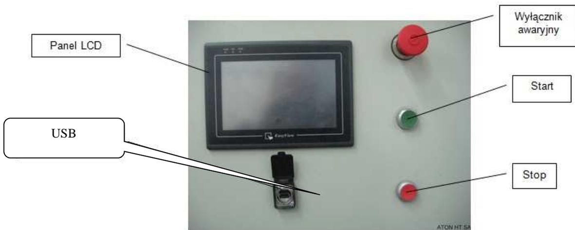
Photo 7. Display on the front panel of the control cabinet
